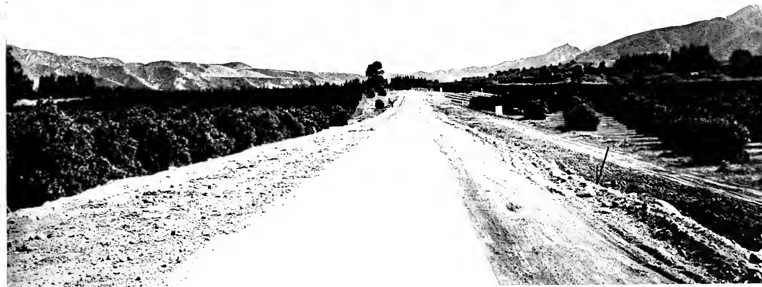
Above pictures show portions of old and new road on realignment of a State Highway lateral eliminating curves between Castaic and Ventura
